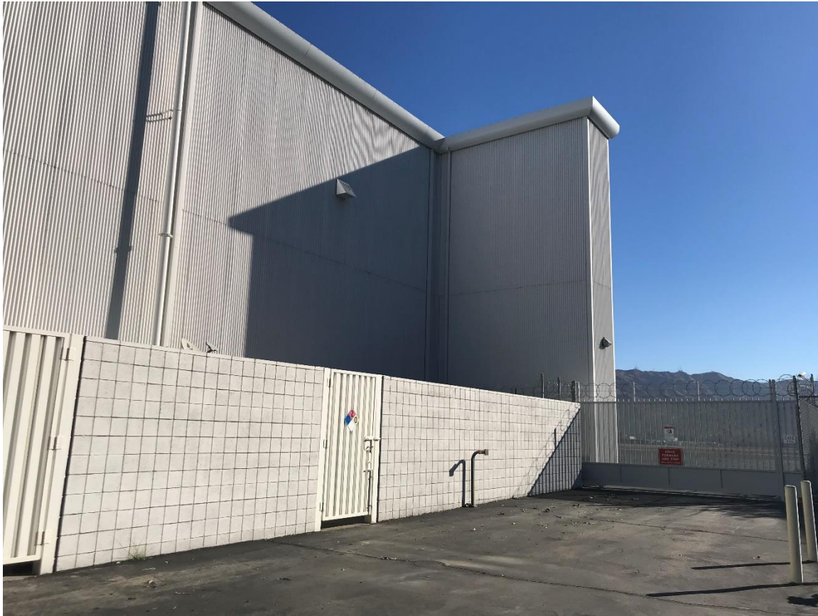
Figure 84 South Elevation of Hangar 22, View East. Towards the center of the image is shown the extension of the front façade, which creates a pocket in which to house the large entry doors that provide access to hangar's interior when they are recessed.
