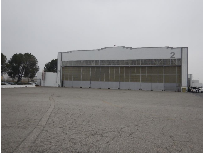
Figure 50 Detail view of East elevation of Hangar 2 showing the large steel multi-glass-paned sliding doors known as “Fenestra Airplane Hangar Doors”
