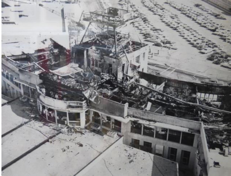
Figure 26 A view of the rear façade of the Terminal Building shows the extent of the damage from the fire, which destroyed the control tower and second floor spaces, including the "Skyroom," photo circa 1966.
