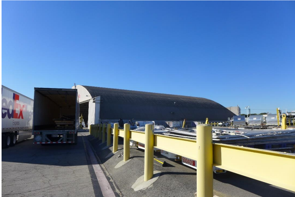
Figure 72 North elevation of Hangar 4 showing Quonset roof, View south
