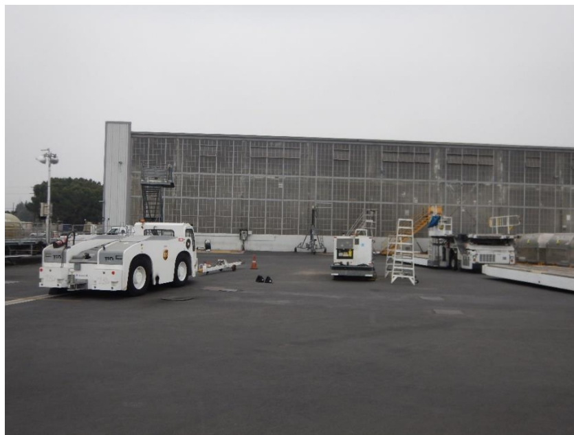
Figure 51 North elevation of Hangar 2 (view south) showing the industrial style windows that exist on each of the side (north and south) elevations of both Hangars 1 and 2
