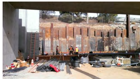
A soldier pile wall supports adjacent land during construction.
